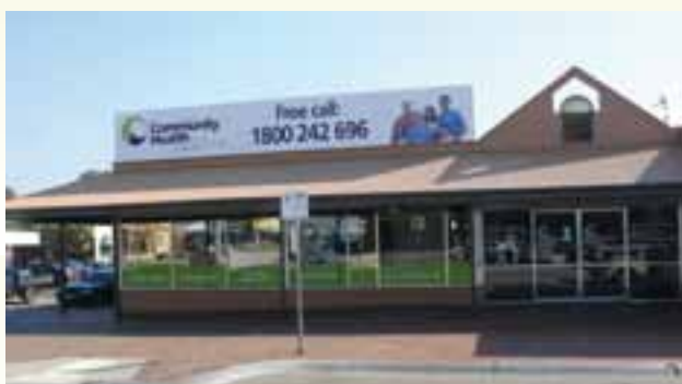
The newly developed LCHS facility in Macleod Street, Bairnsdale.
