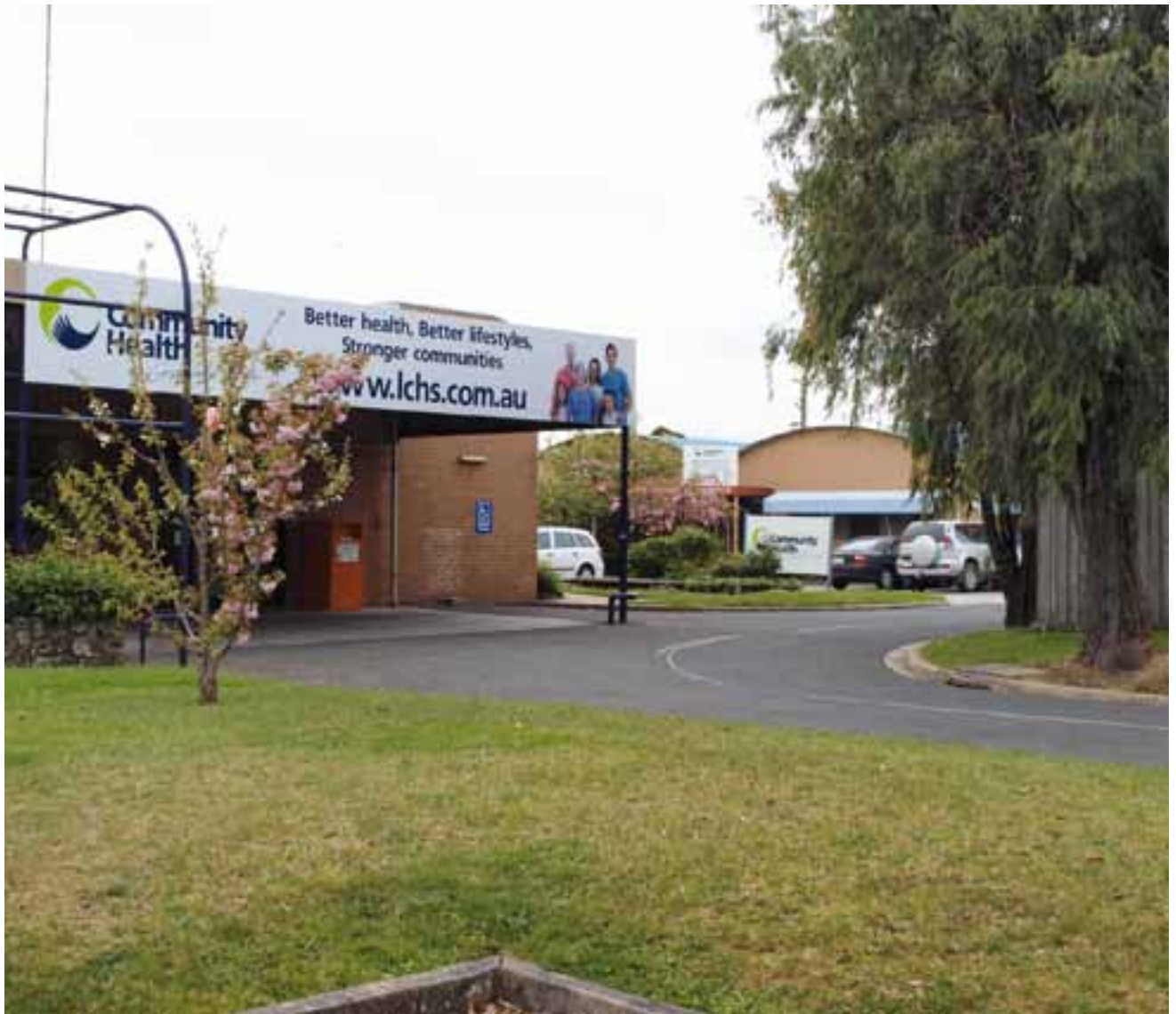
The re-branding program was finalised with the installation of new signage at Moe (above and top left).
