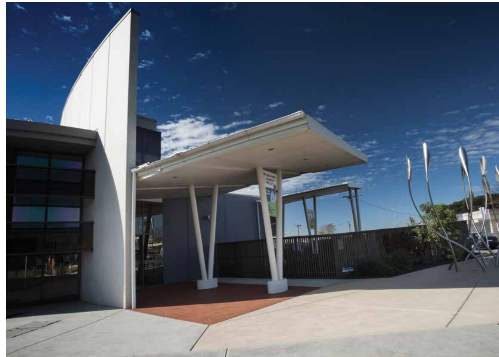
Latrobe Community Health Service Morwell office.
